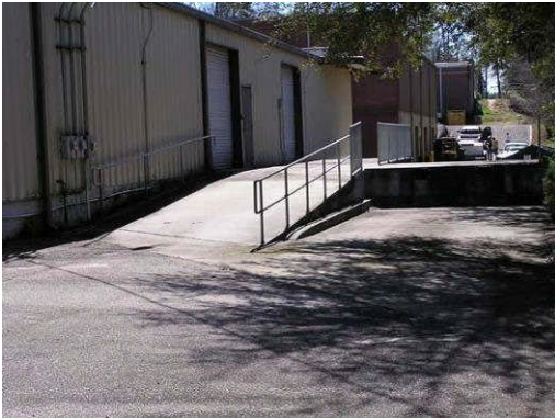
Fig. 10: A slope at the back of a warehouse.
